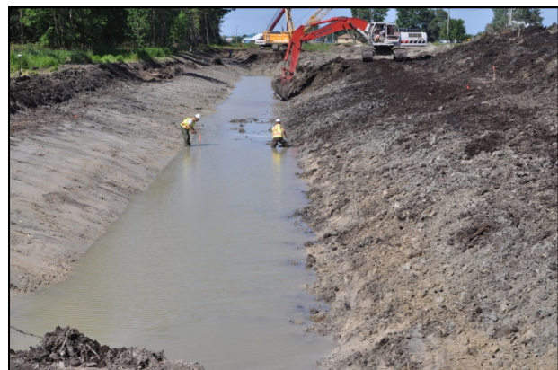
Construction of the Canal
